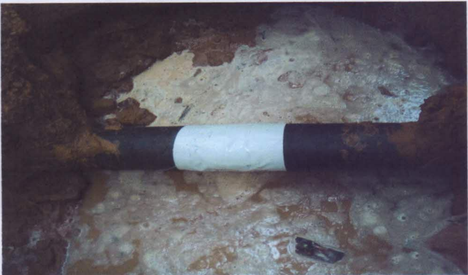
Fig C: picture taken after repairs
