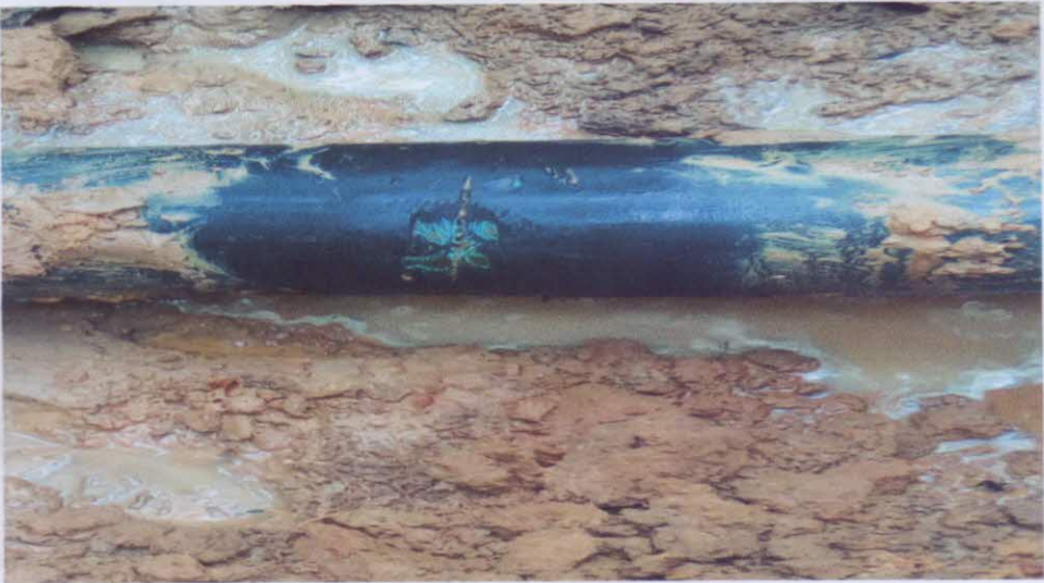
Fig A: picture taken after excavation.
